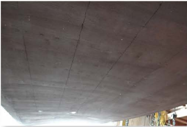
This 10-year old 'shortcut' 5200 bottom had never been put in the water. 24-tubes of rubber were billed and no CPES or barrier coat primer. Note how plank shrinkage cracked seams and left bung putty proud.
