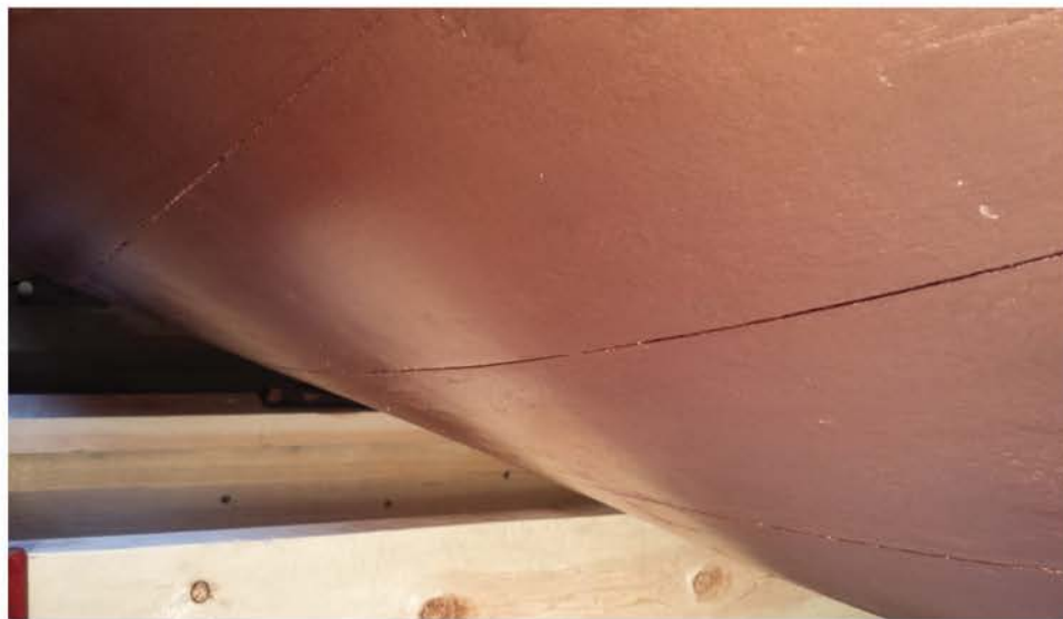
A well-used, 10-year old 'shortcut' 5200 bottom showing open seams. The owner was billed for 24-tubes of 5200, obviously not enough. Also, no barrier coat primer.
